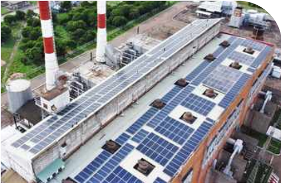
Rooftop solar power project in Thu Duc - 524kWp Location: Ho Chi Minh
