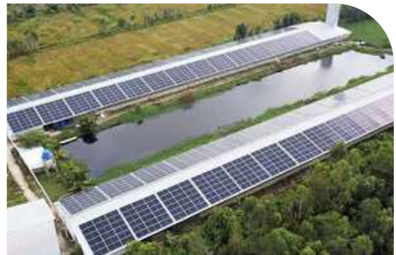
Rooftop solar power project at Tu Huu Farm - 534.24 kWp Location: Kien Giang
